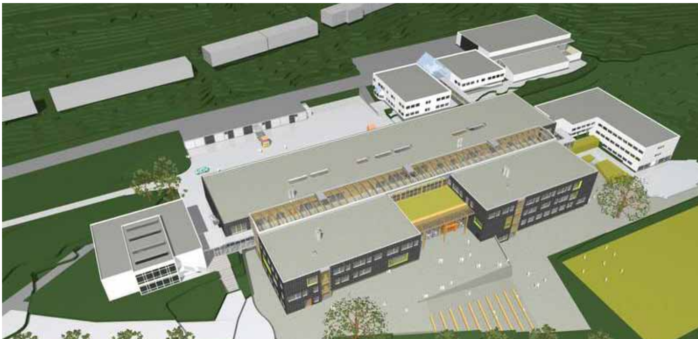
Betonmast: Romsdal Videregående Skole
